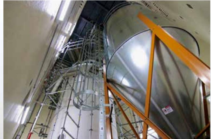
Figure 6. CSSF 1 nested bin replica and storage vessel.
