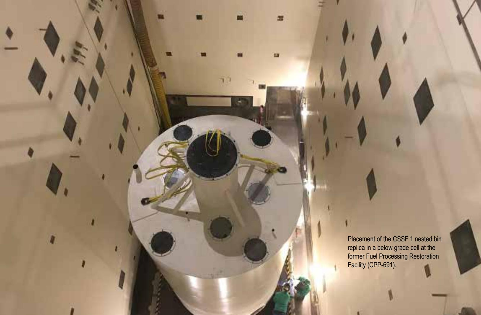
Placement of the CSSF 1 nested bin replica in a below grade cell at the former Fuel Processing Restoration Facility (CPP-691).
